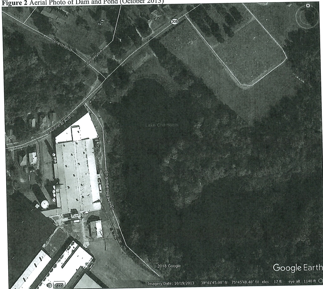
Figure 2 Aerial Photo of Dam and Pond (October 2013)
