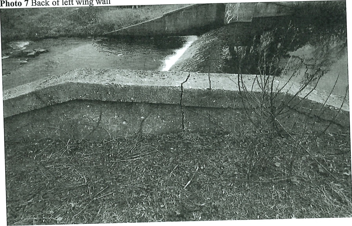
Photo 7 Back of left wing wall
